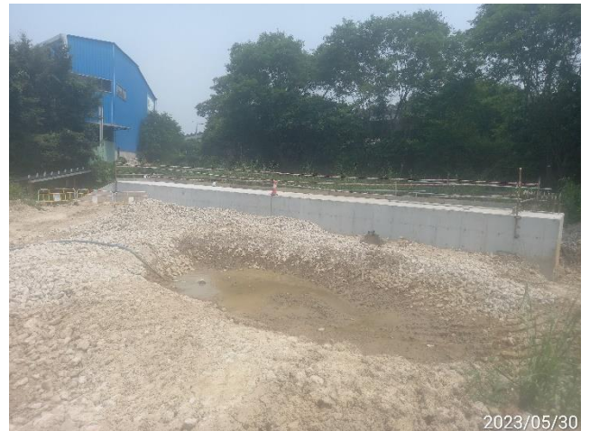
Sump formed next to the finished box culvert (R2)
