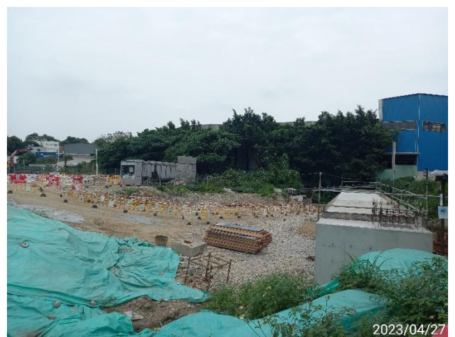
Works area near the box culvert (R2)
