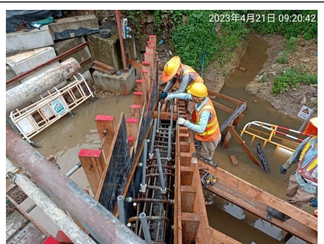
Works at the box culvert (R2)
