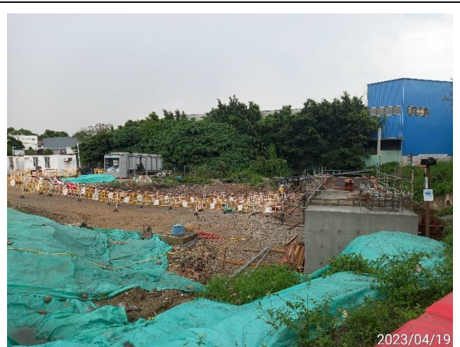
Works area near the box culvert (R2)
