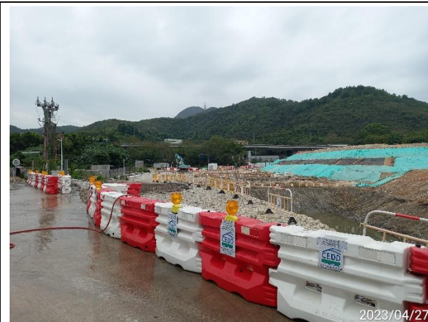
Works area next to the access road/ Site 3-8 (R1)
