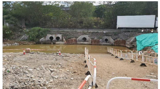
Wastewater was diverted to sump pit. No discharge of wastewater offsite was observed during site investigation.
